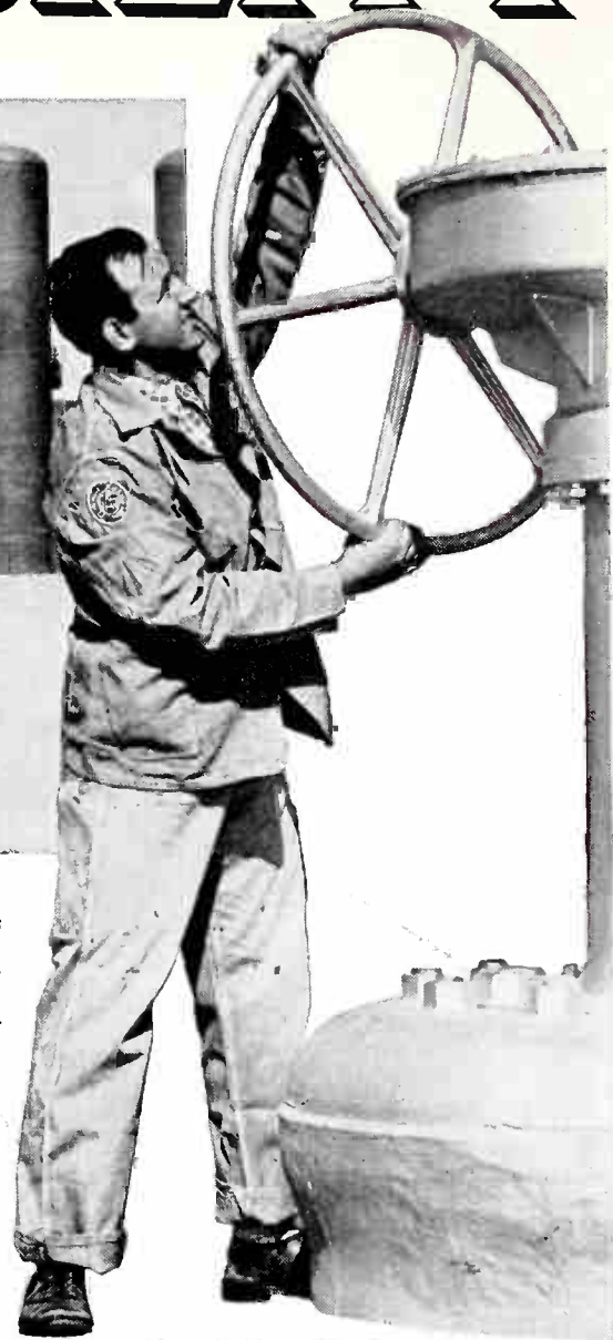
(Right) Receiving natural gas by pipeline from southwestern states, Michigan Gas stores it underground in depleted wells converted for the purpose.
